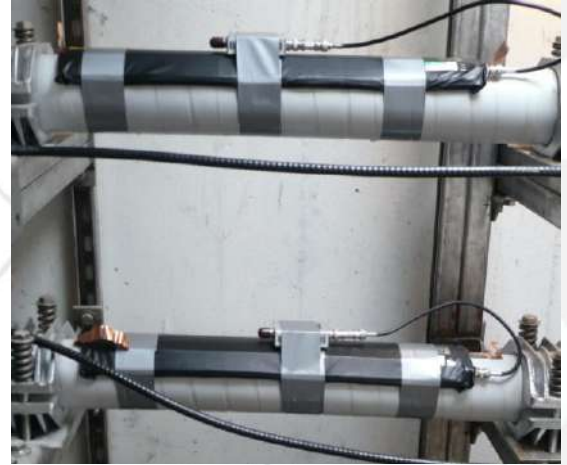
Example of FMC on high voltage cable Standard installation on HV cable, with Amplifier
