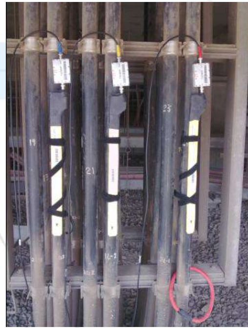
Example of FMC on medium voltage cables
